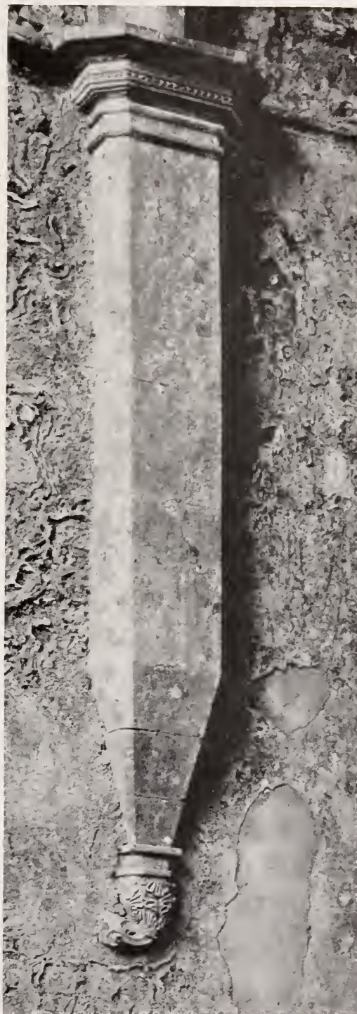
VAULTING-SHAFT IN CHANCEL ABBAY KNOCKMOY
