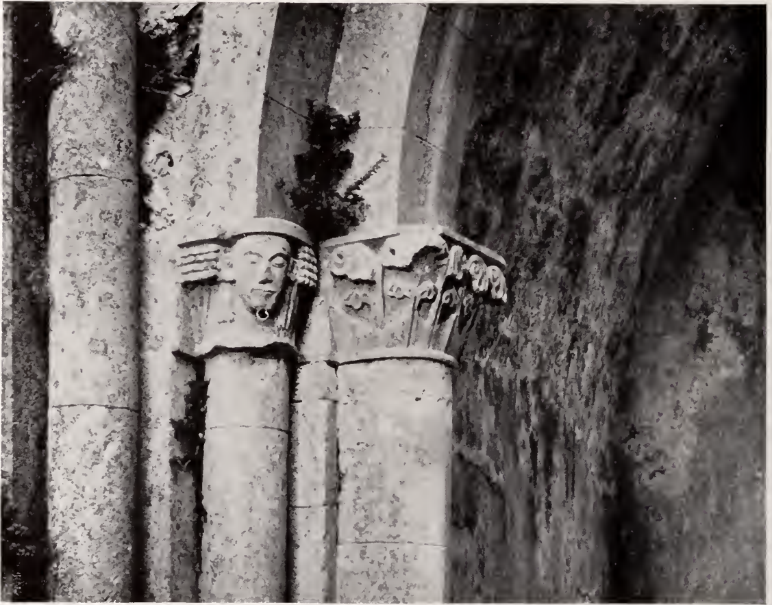
CAPITALS AT ENTRANCE TO SOUTH TRANSEPT CHAPEL, CORCOMROE ABBEY
