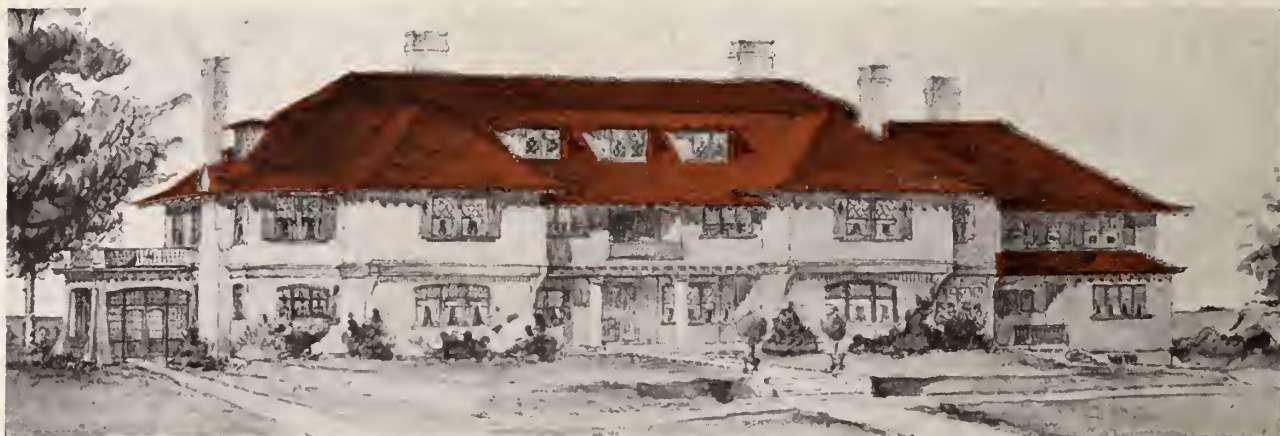
House under course of construction at East Brewster, Mass., for Mrs. Roland C. Nickerson.
