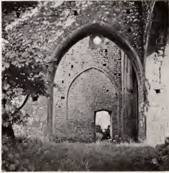
HORE ABBEY, VIEW ACROSS EASTERN BAY OF NAVE
