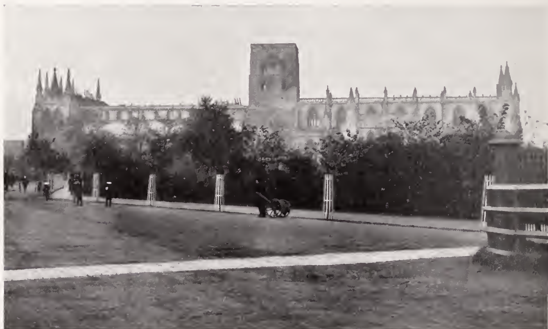
VIEW OF SOUTH SIDE AFTER THE FIRE
