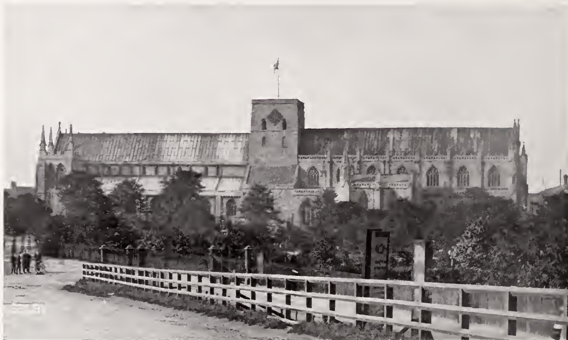
SOUTH VIEW, BEFORE THE FIRE
