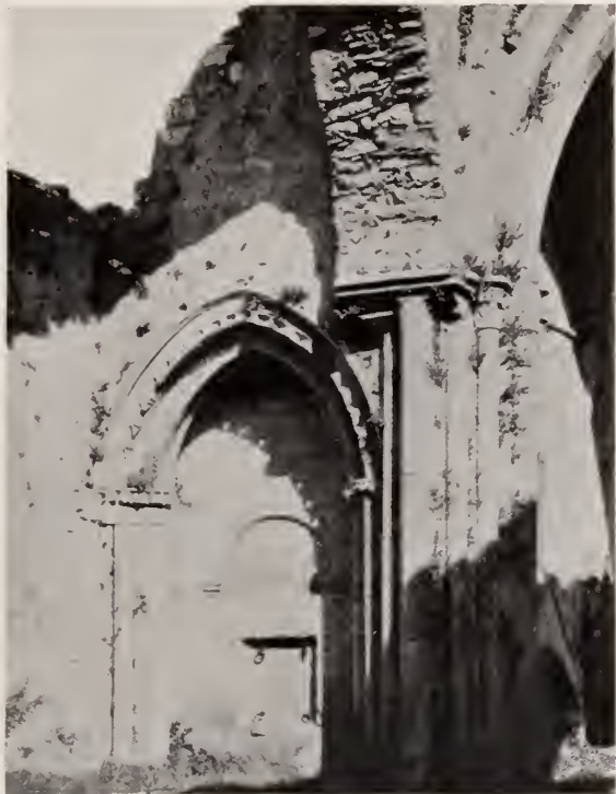
DOORWAY WITH THIRTEENTH CENTURY BILLET, CASHEL CATHEDRAL
