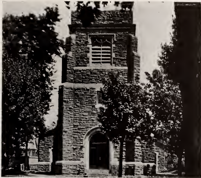
ST. PHILIP'S CHURCH, DURHAM, N. C. CRAM, GOODHUE & FERGUSON, ARCHITECTS ALL TRIM AND TRACERY IN CONCRETE STONE BY ECONOMY MANUFACTURING COMPANY, NEW HAVEN, CONN.
