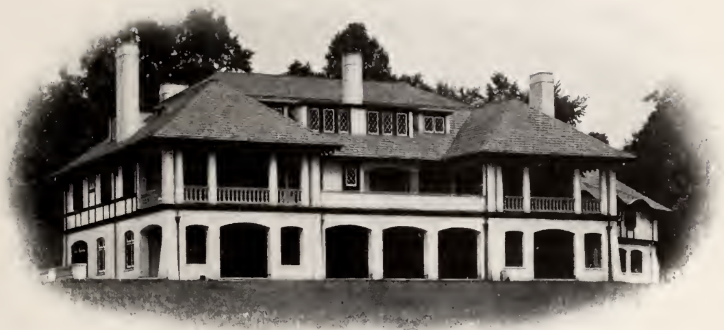
Residence of Mr. W. Plunkett Stewart, at Haverford, Pa. Chapman & Frazer, Architects
