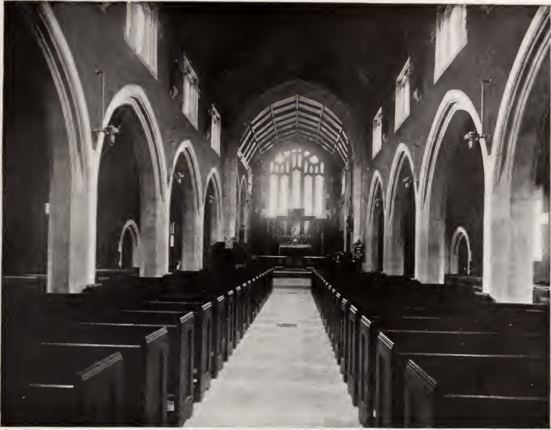
INTERIOR OF CHRIST CHURCH, WEST HAVEN, CONNECTICUT
